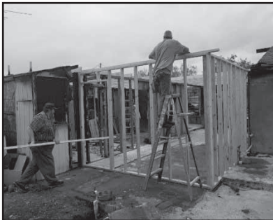
Repairing Maria Ayala's home.
